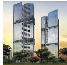
Echelon Tower Singapore Construction period: 2013–2016
